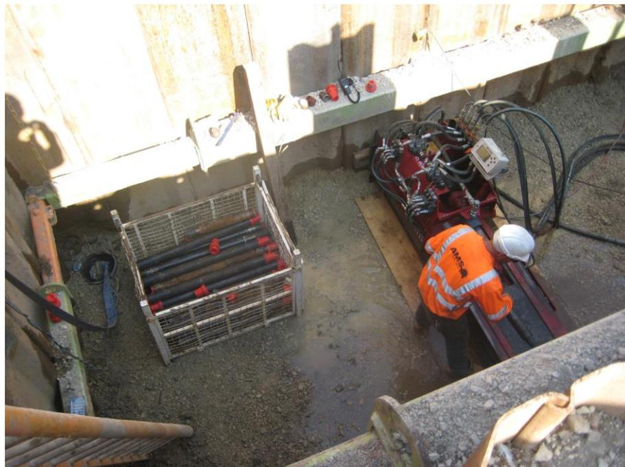
*AMS No-Dig's Pit Launch directional drilling rig in place ready to start drilling*
