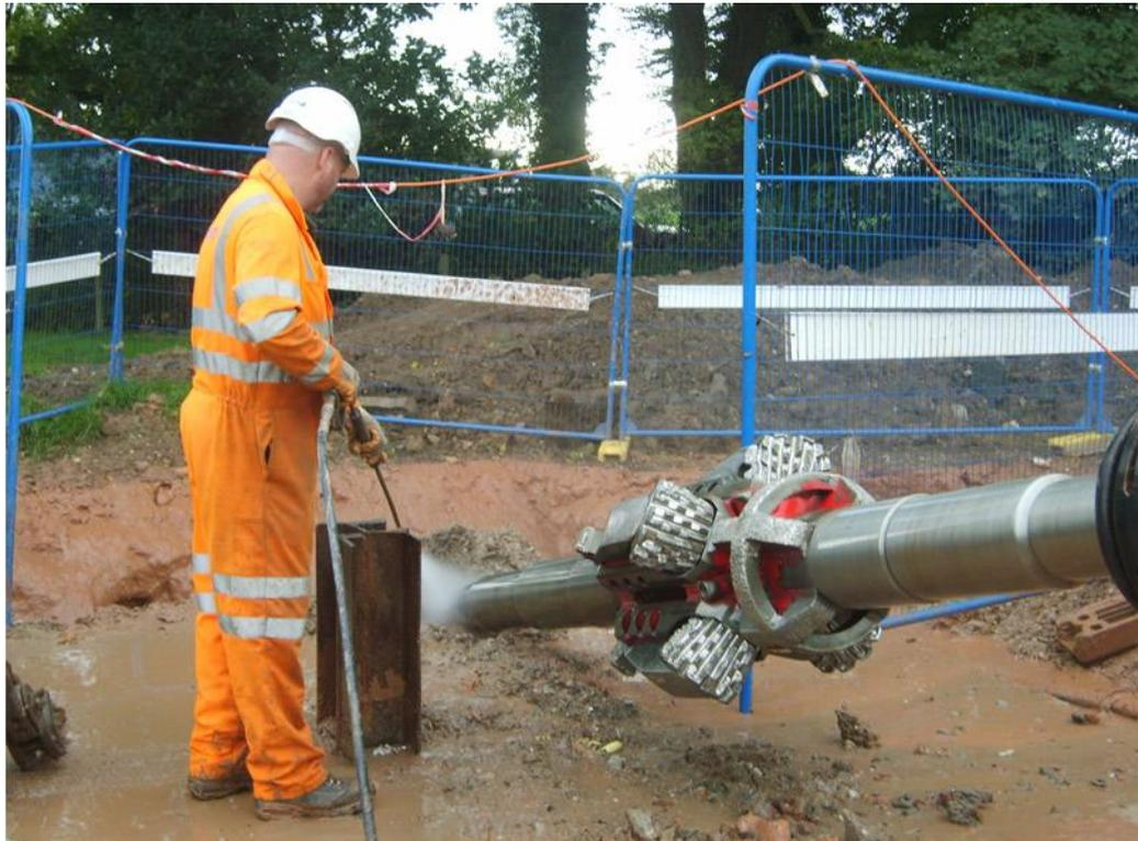
*R17 hole opener fitted with 22inch rollers*
