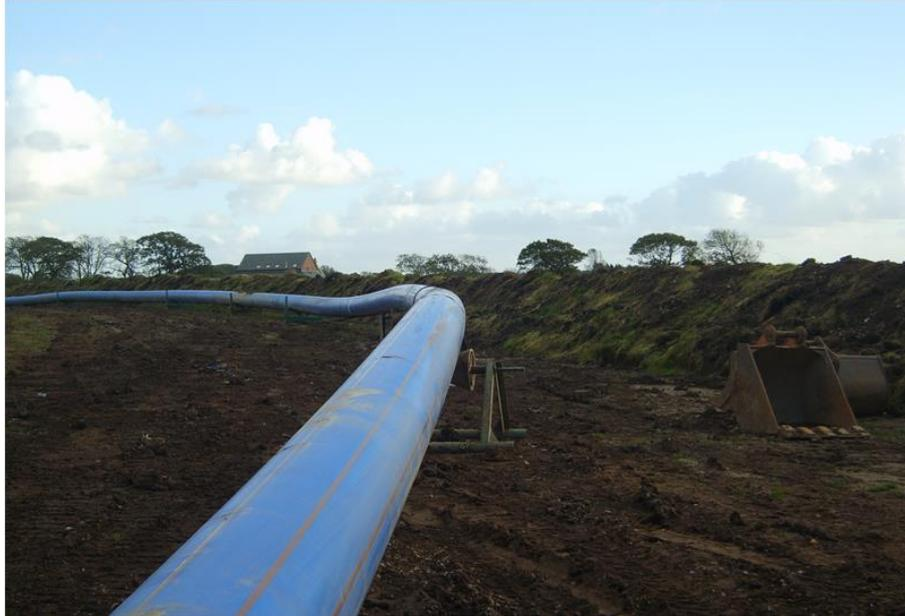
*630mm HPPE pipe on low friction rollers ready for installation*
