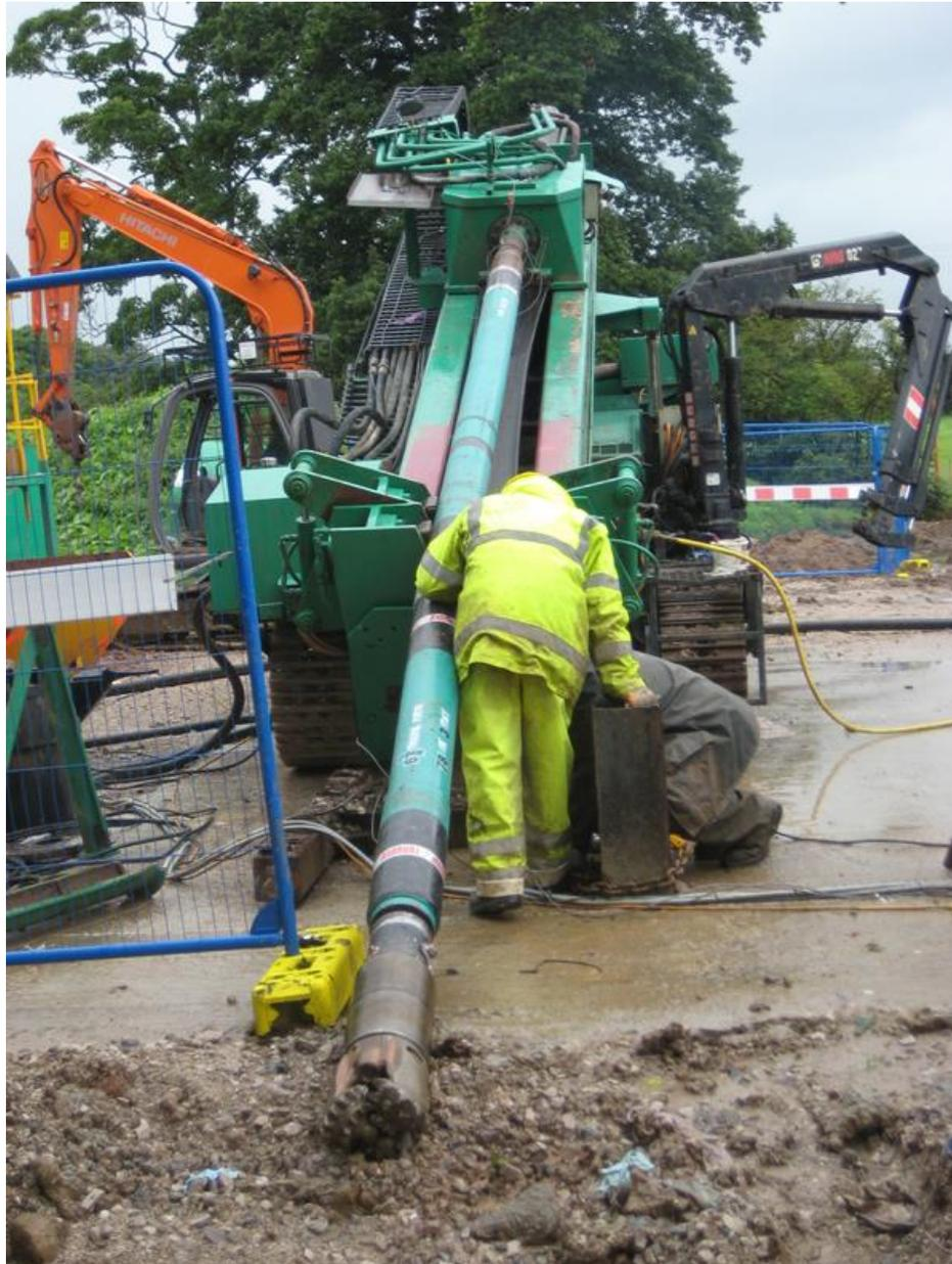
*6.75 inch mud motor fitted with 9.87 inch tricone bit*
